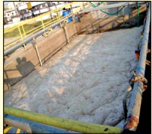
Biological Treatment (SBR)
